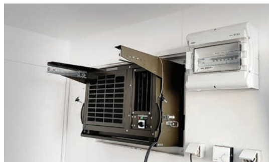
Container installation - inside view
