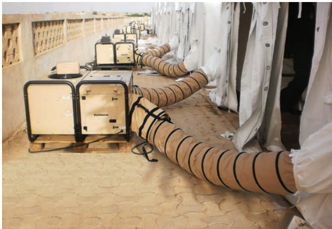
Installation with the air ducts
